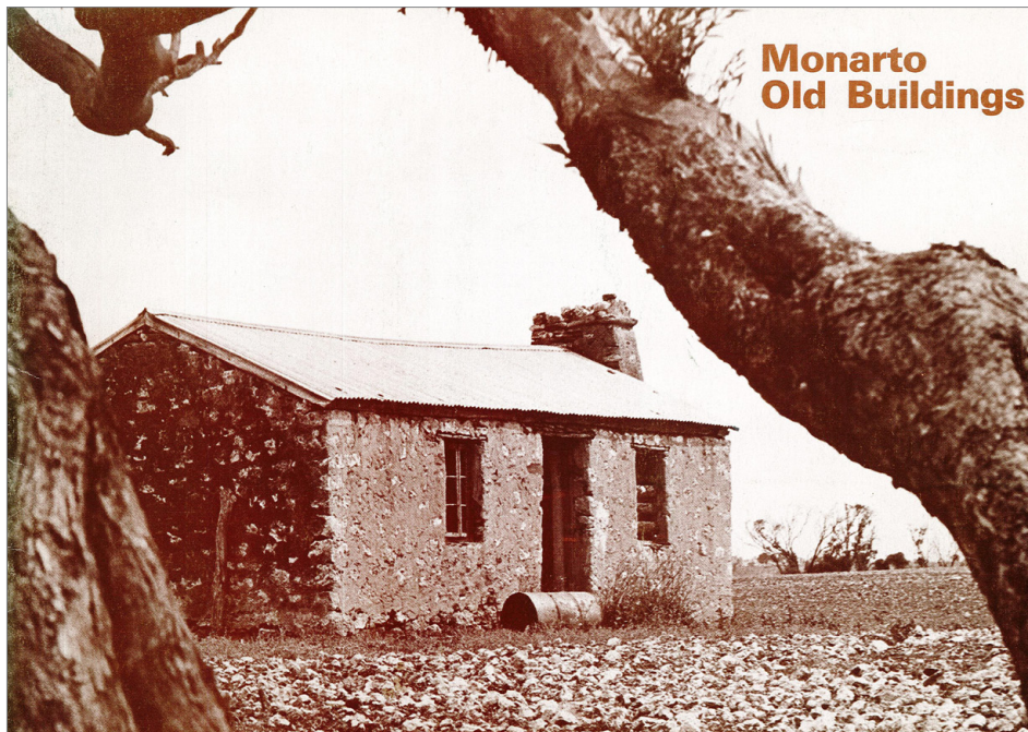
Figure 4: Front cover of the Monarto Old Buildings report. (Monarto Development Commission, December 1974.)
