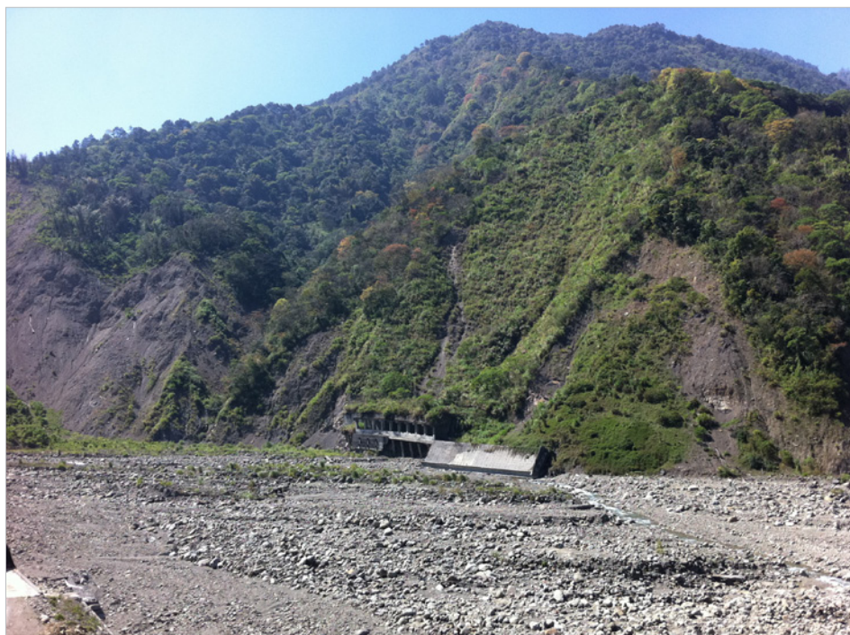
Figure 8: On any days with heavy rain, landslides and mudslides of the Shenmu village might destroy roads and bridges. Villagers, therefore, have developed their own 'do-it-ourselves' rescue plan.
