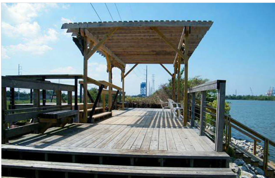
Figure 12: Completed and repaired platform, bayou side, 2011.
