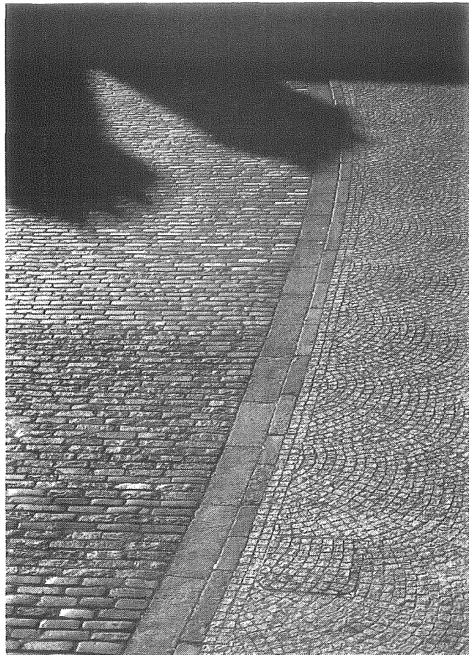
Figure 2: Upper Castlehill, Stirling. New and recycled stone elements are used together
