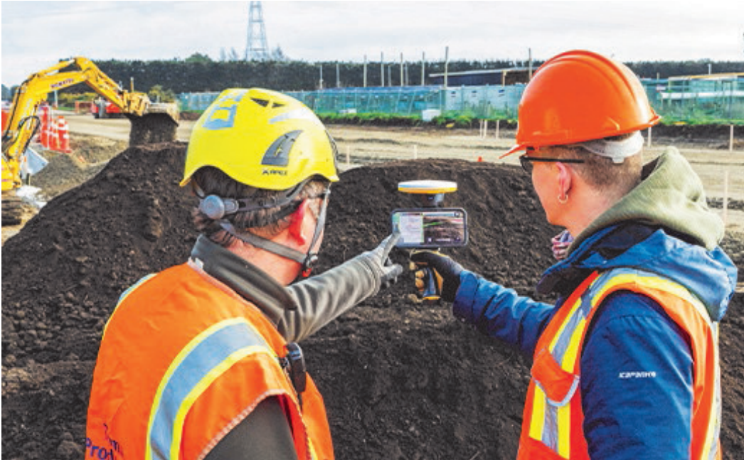
Figure 4. Construction workers using Trimble SiteVision to view digital site information in its real-world context (Trimble SiteVision product page, retrieved 2026).
