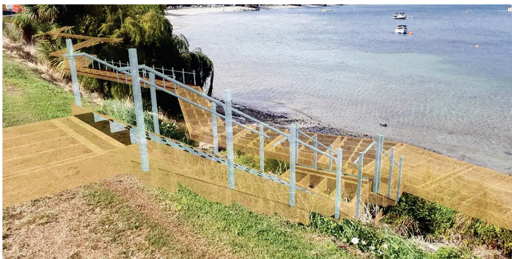
Figure 1. Timber framing for designed boardwalk at Lake Wanaka (with permission from Blakely Construction, February 2021).
