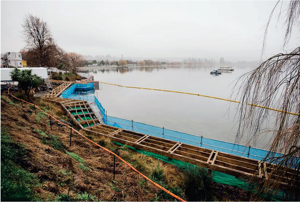
Figure 2. Boardwalk under construction at Lake Wanaka (with permission from Blakely Construction, June 2021).
