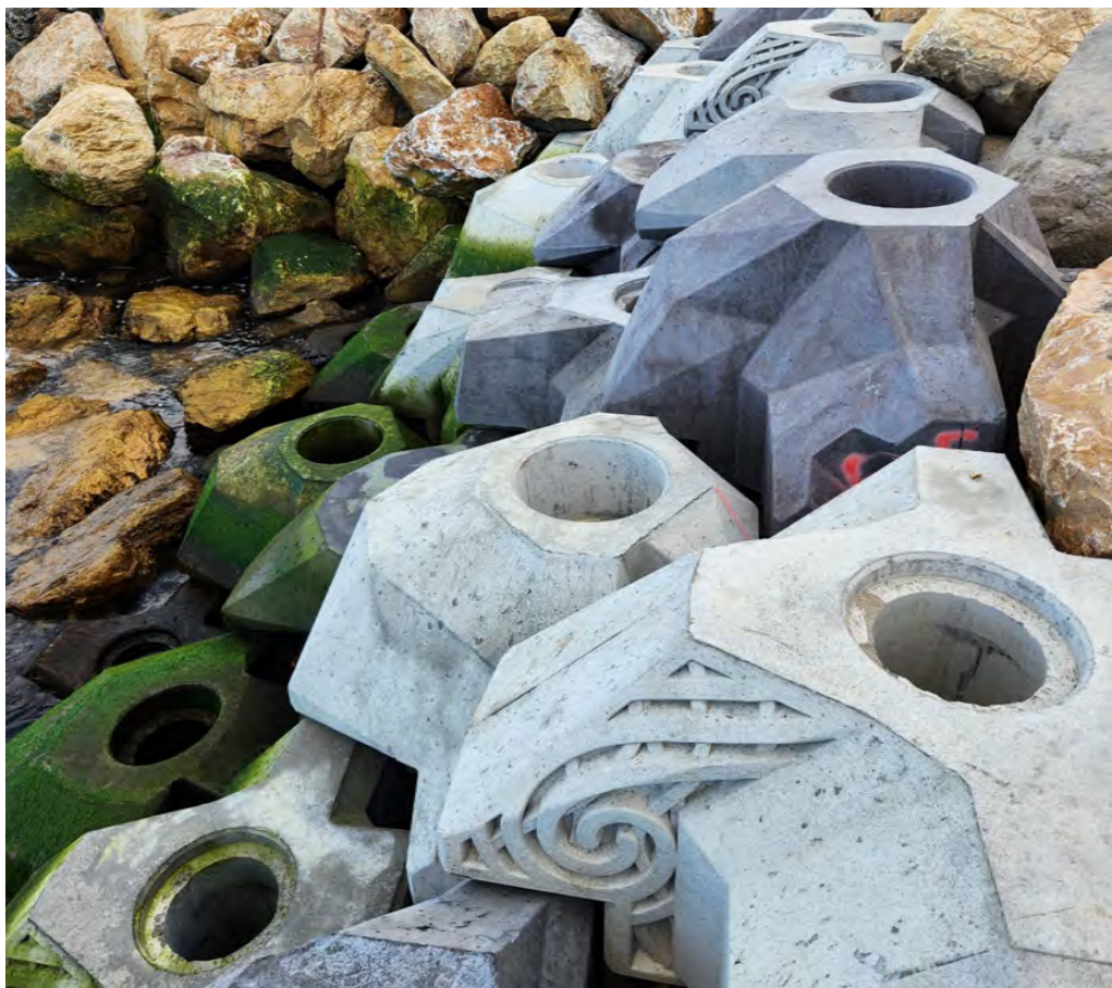
Figure 10. Ecological Xblocs integrated with cultural artwork. While functionally above the tide, the artwork provides an important conceptual link between sea and land for mana whenua (image by author, August 2024).
