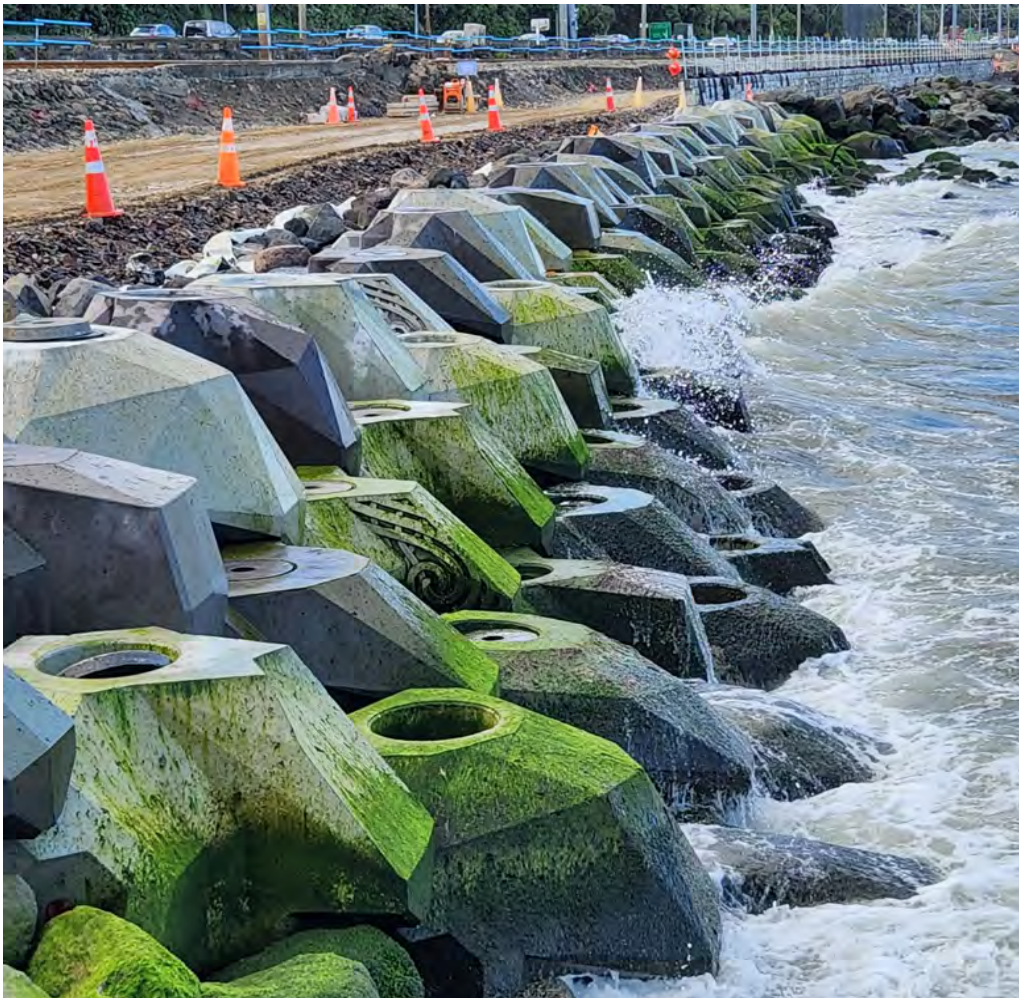
Figure 6. View north. Transport corridor to top left. Architectural and ecological Xblocs, both modified from the original functional Xbloc exhibiting initial algal growth after recent installation. The northern end of the project is shallow compared with the southern end (image by author, August 2024).
