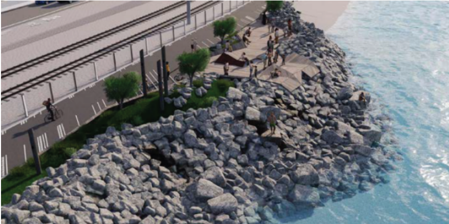
Figure 7. Example of an ūrangā (buildout) with accent rocks. Note ūrangā revetments are constructed of rock rather than modified Xbloccs. The latter are used to support the path (along with seawall sections) between ūrangā (with permission from Isthmus, August 2024).
