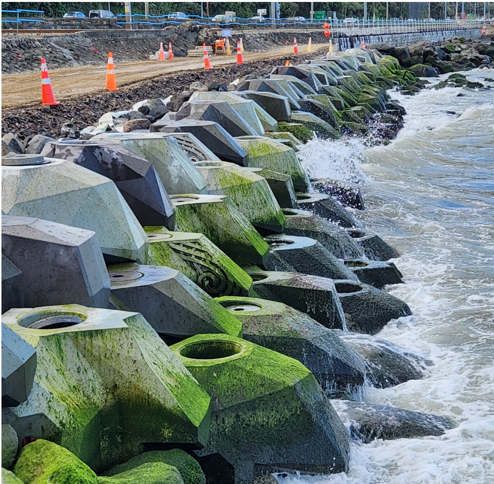
Figure 6. View north. Transport corridor to top left. Architectural and ecological Xbloccs, both modified from the original functional Xblocc exhibiting initial algal growth after recent installation. The northern end of the project is shallow compared with the southern end (image by author, August 2024).
