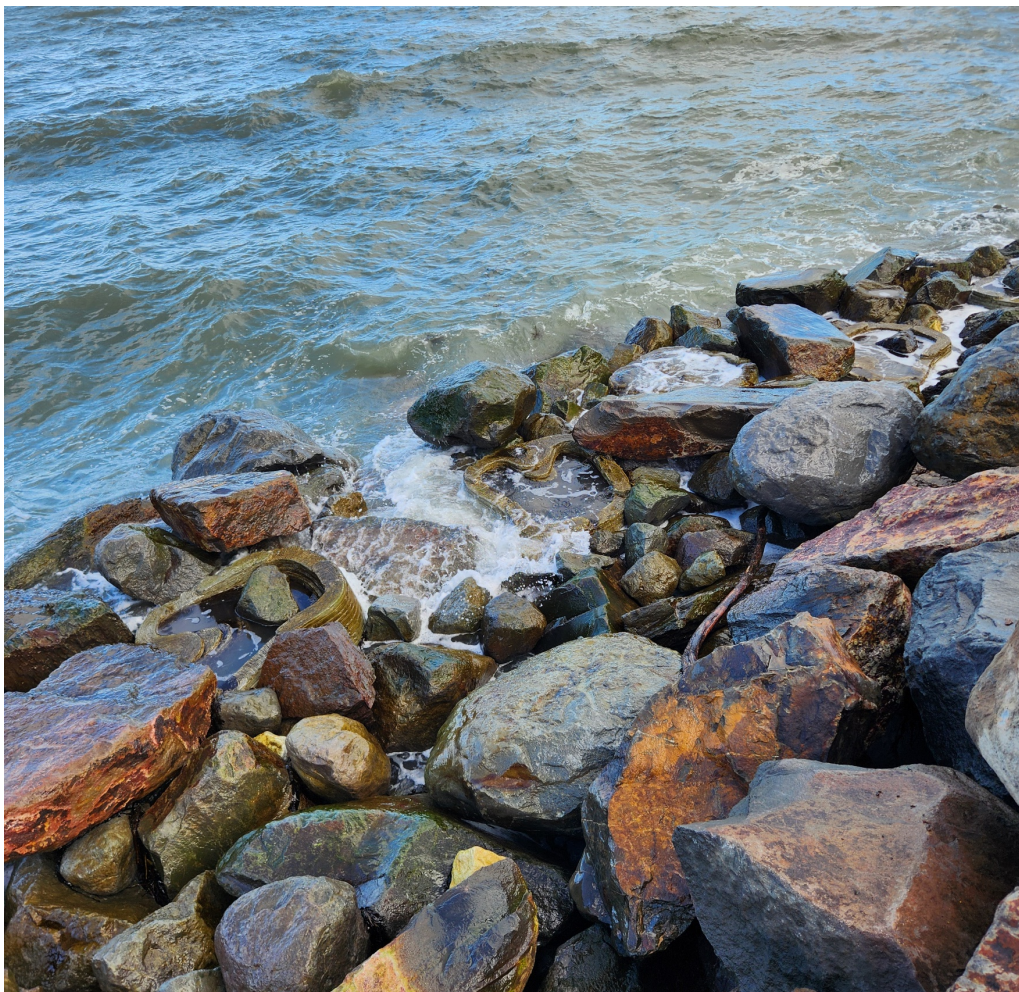
Figure 11. Construction phase. Tide pools required for ecological mitigation provide variability, enrich experience and exhibit a duty of care to build back opportunities for life (image by author, August 2024).
