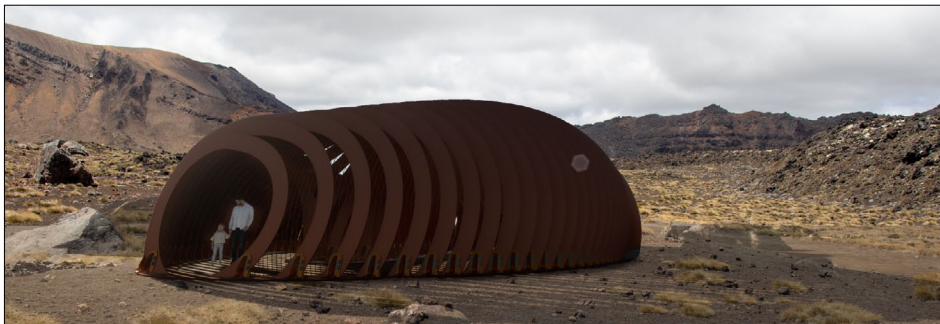
Figure 8: The wharepaku unit sits on the surface so no digging on the maunga is required.
