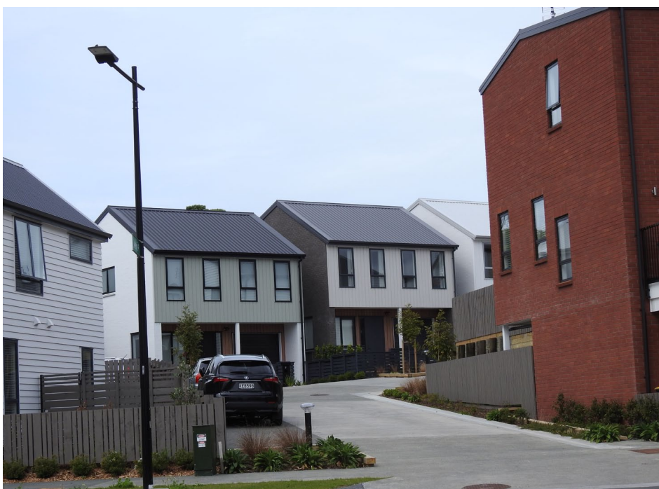
Figure 6: Recent urban renewal in the Fenchurch Street area of Glen Innes, November 2020. Buildings include state rental, private rental and affordable (to some) homes. (Photo: Diane Menzies.)
