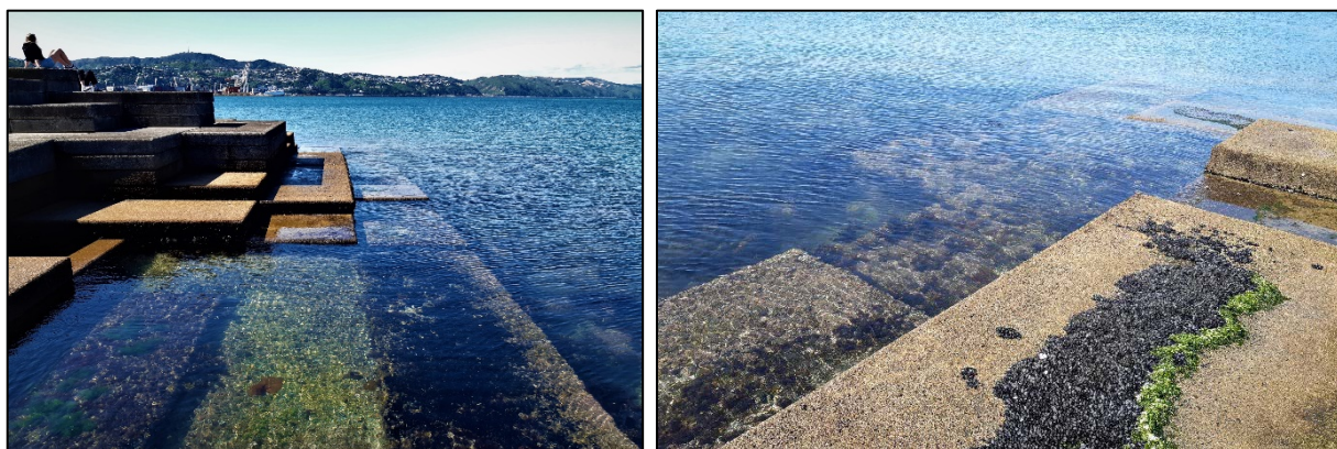
Figure 13. Oriental Bay Enhancement by Architecture Workshop in Wellington Harbour in New Zealand. People use this urban designed public space for contemplation and interaction with the sea. The design of the structure incorporated the transient nature of the tides through the use of steps, rock reefs and intertidal pools, allowing people to see and touch the marine lifeforms. Image credit: The photos were taken by the author in December 2019.
