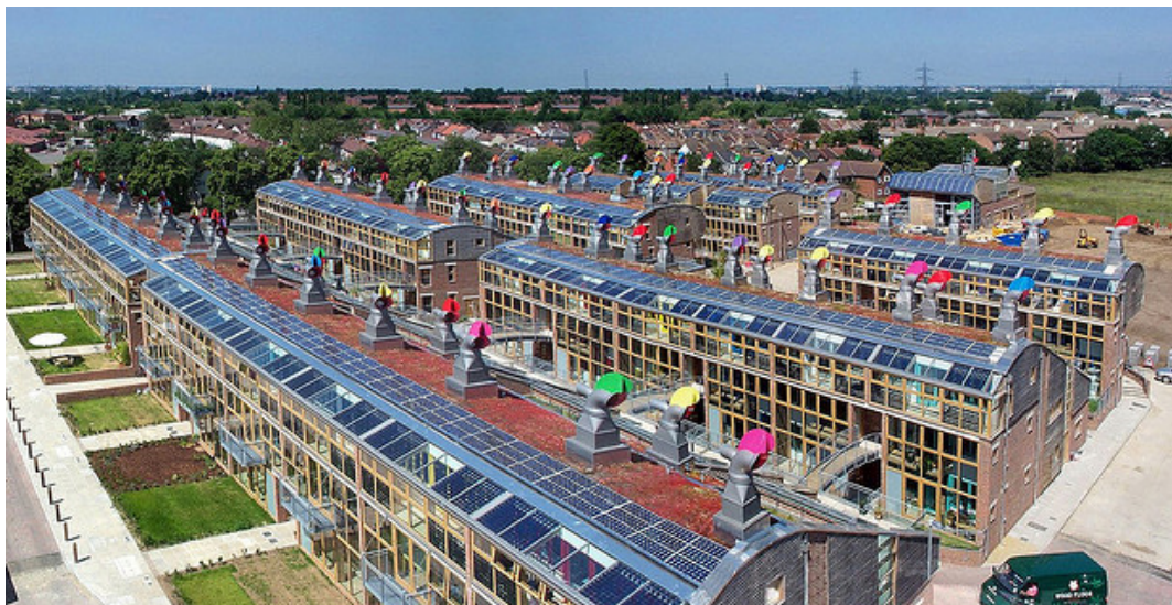
Figure 2: BedZED, London, UK Source: ( http://www.peabody.org.uk/mediacentre/casestudies/bedzed.aspx )
