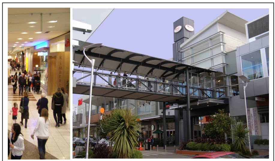
Figure 6: Pedestrian arcades and covered walkways at first floor level Source: E G Pryor
