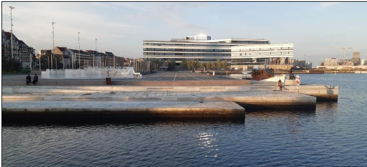
Figure 3: A typical form of urban coastal harbour edge condition with a defined, segregated, hard boundary between land and water that severs a closer and more tactile connection with the water and its life forms. The public space in the waterfront is mainly is made of concrete for humans. Very little consideration is given to terrestrial plants, and there is no designated space for interacting with the marine world. The photo was taken by the author in Aarhus, Denmark, in October 2021.
